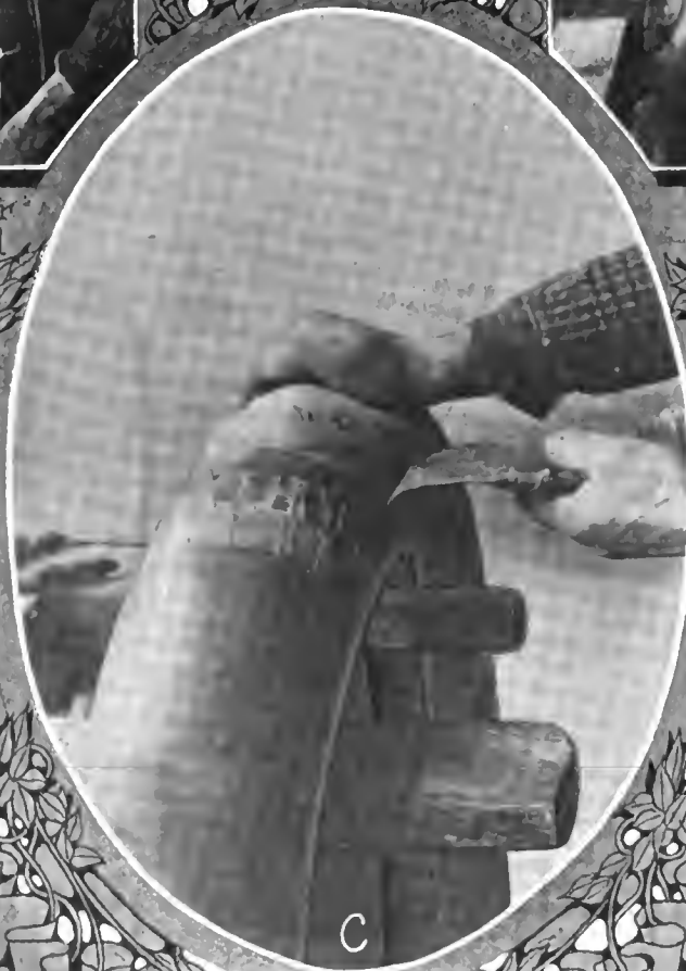
Stripping Canvas from Section to be Repaired
